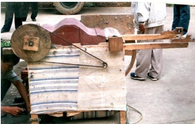
Installing the shredding machine
